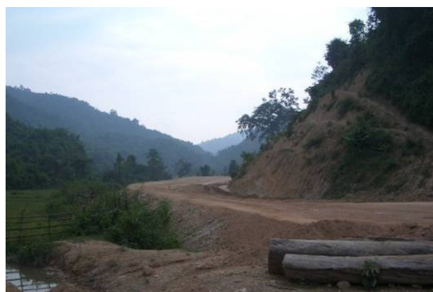
Figure 8: The construction of R3E
